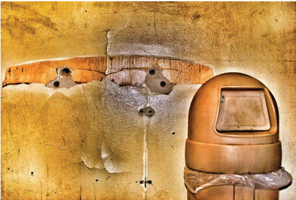
Hallway wall, Elementary School No. 20, Paterson.
