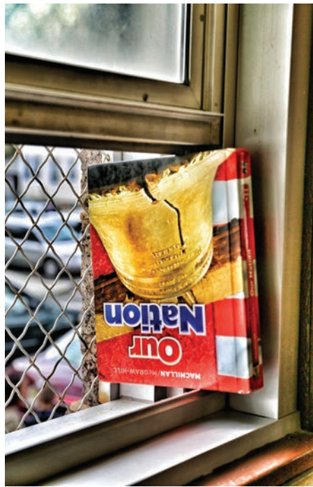
Broken window in an in-use classroom, Elementary School No. 20, Paterson.
