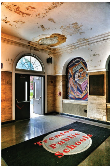
Main entrance, Trenton Central High School
