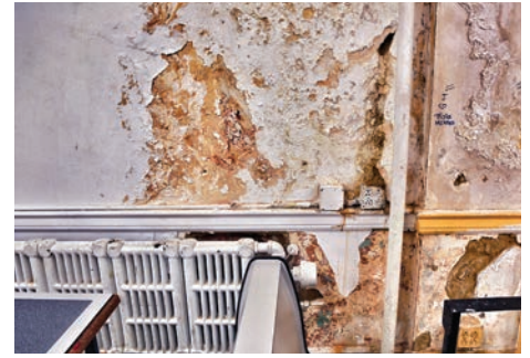
Trenton Central High School cafeteria.
